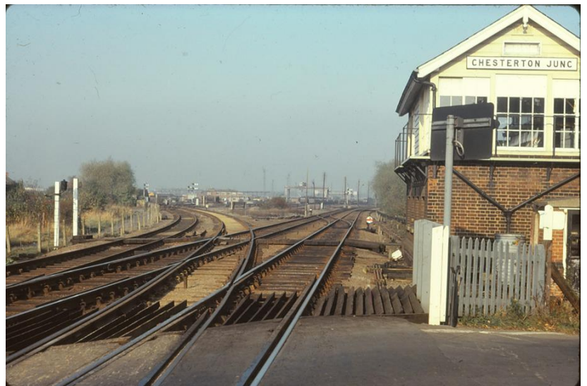
Chesterton Junction 1975. The short-lived (1850) station probably lay in the angle between the main line to Ely (right) and the St Ives branch (left). (Tony Kirby)
